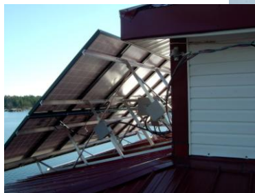
Commissioning 20 K.W. SMA ® system (4-5000 W inverters stacked)
