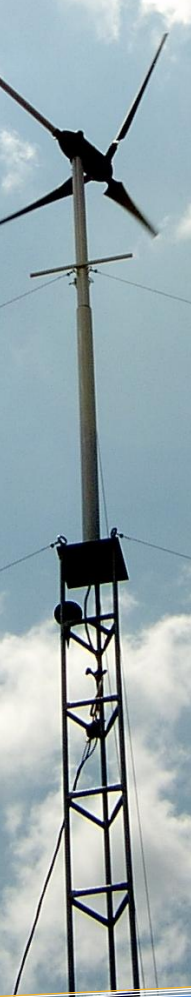
Commissioning 20 K.W. SMA ® system (4-5000 W inverters stacked)
