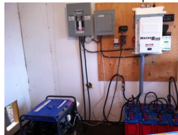
Magnum ® MS4024PAE system with auto gen start to propane powered generator
