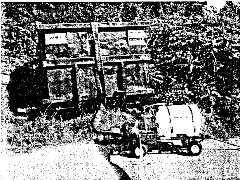
Photo's #11. Examples of our patented inline de-chlorination system, low boy dumpster bucket which has a sediment geo-bag connected to the drain hose inside the dumpster bucket. After the sediment removal process the dumpster is removed from site and taken to landfill.
